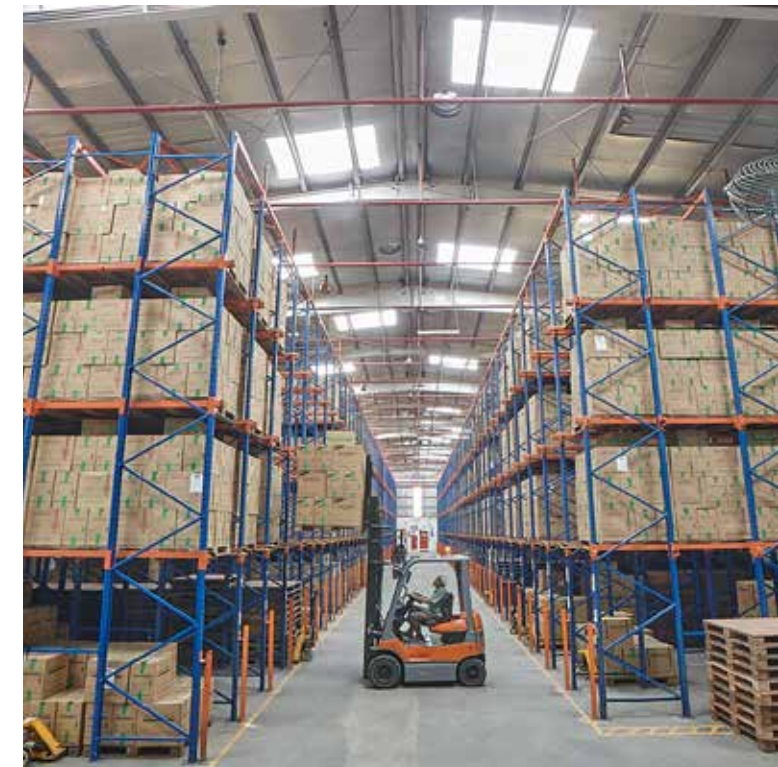
Prismatic skylight in the factory to reduce electricity consumption
