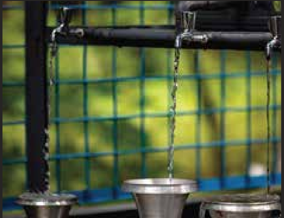
Stream of Pure Drinking Water from Probaho Water Filtration Plant, Jhenaidah
